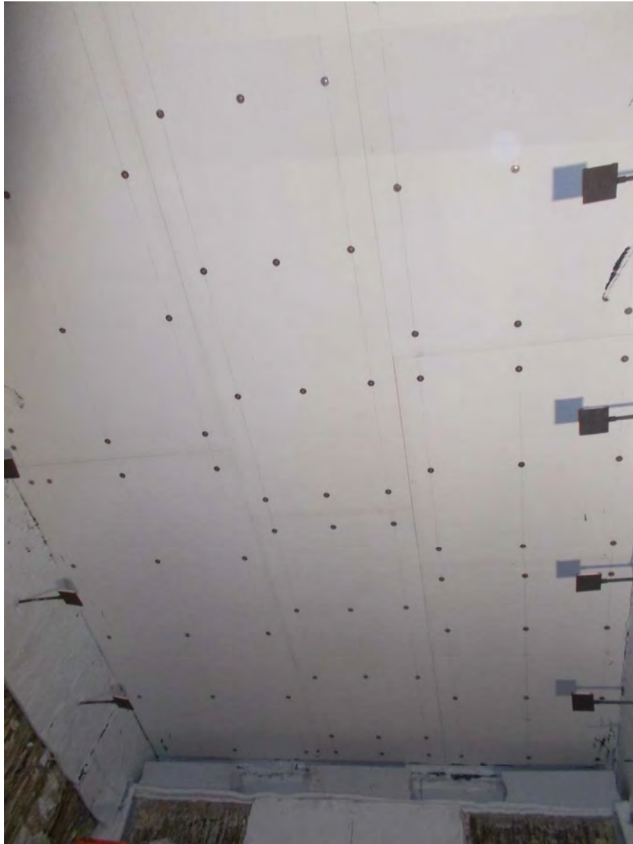
Photo K Exposed side before the start of the test.
